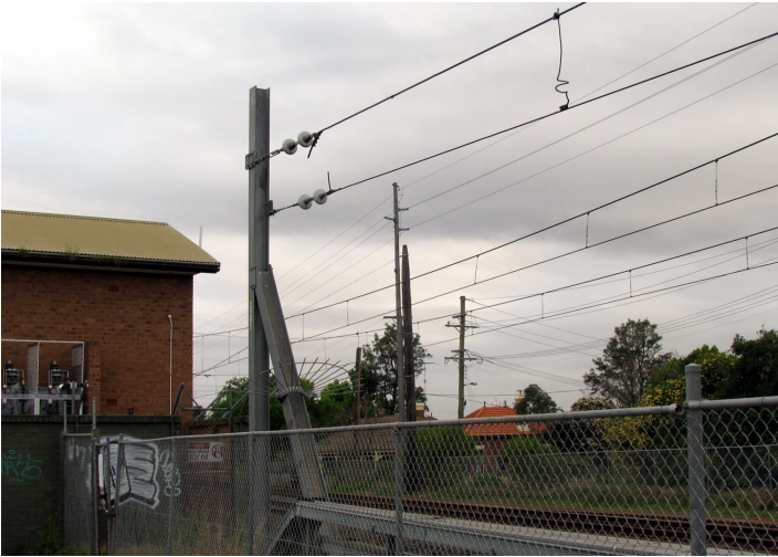
Example of a Fixed Termination Mast and Traction Substation.
