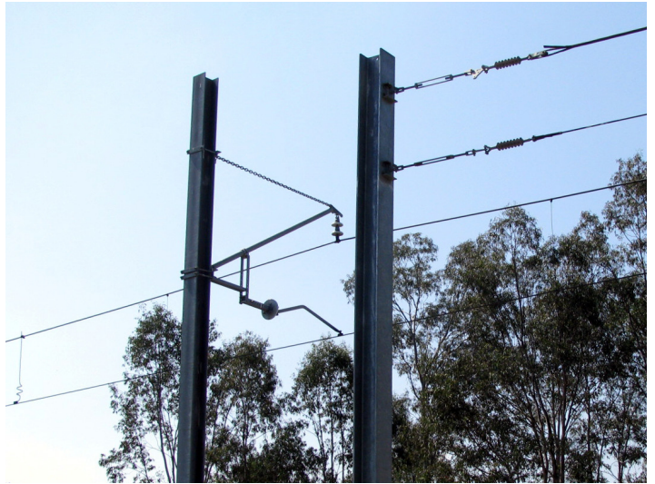
Example of a Fixed Termination Mast.
