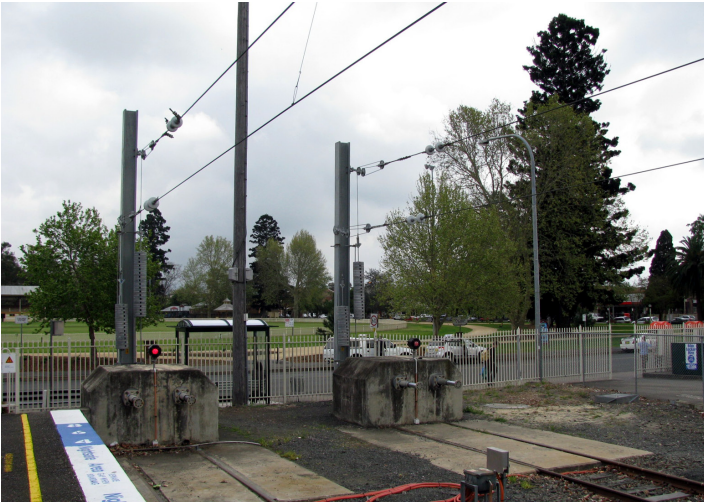
Example of a Termination Spanner.
