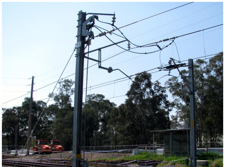
Example of a Feeder Mast.
