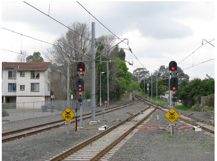
Example of a Double Bracket Mast.
